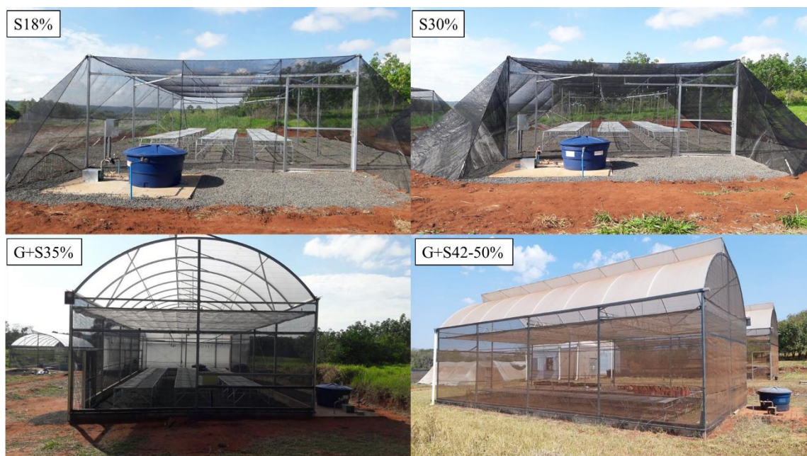
Fig. 1. Environments: S18%: screenhouse with 18% shading; S30%: screenhouse with 30% shading; G+S35%: greenhouse + Aluminet® screen with 35% shading under the plastic film; G+S42-50%: greenhouse + Luxinet® screen with 42-50% shading under the plastic film.
