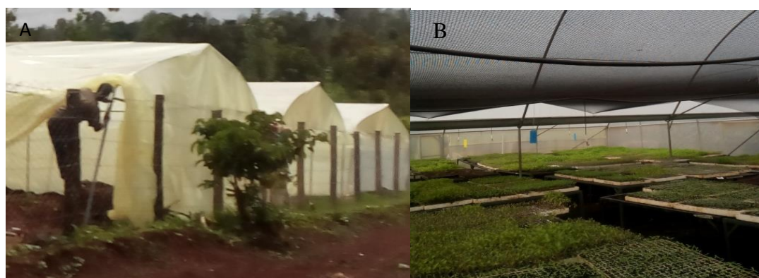
Fig. 6. Greenhouse designs for; A - Locally assembled low tunnel greenhouse, B - Propagation House with misters, (Source: Author designs, 2020).
