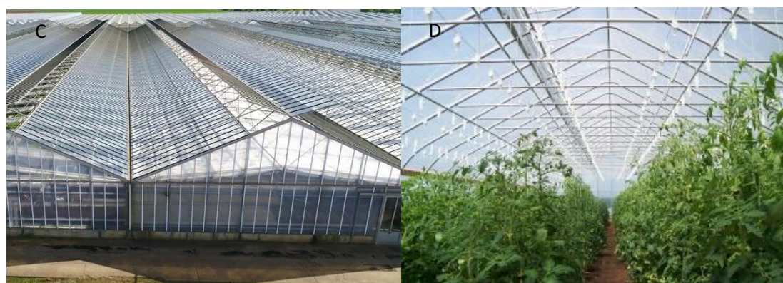
Fig. 7. Greenhouse designs for; C - Extensive multi-arc greenhouse and D High Tunnel - vented and automated greenhouse (Source: Shutterstock.com).
